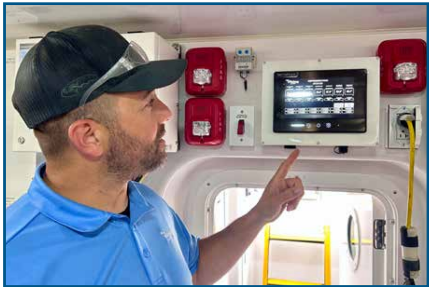
Ryan Jenkins shows the OctoPlex refrigeration screen for monitoring box temperatures.
