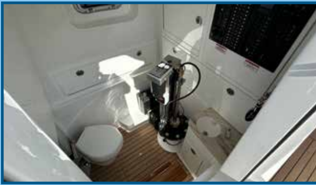
Inside the console, the Simrad SY50 omni sonar – the first installed in a Valhalla 41 – required in-house engineering and custom modifications, including a 3D-printed dam and a reworked console liner.
