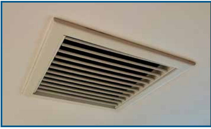
Above: A dehumidification vent aboard the Viking 82 helps control moisture.
